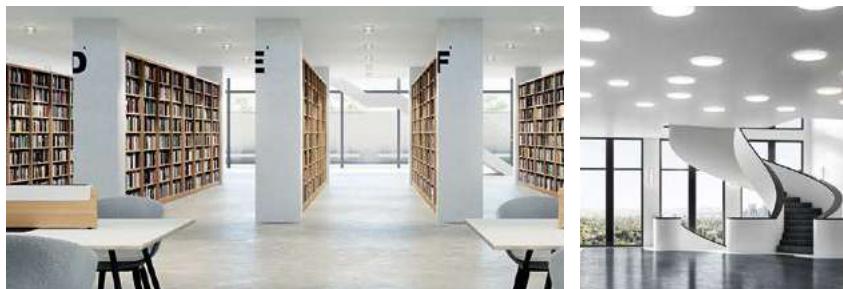
DALI control capability is easily retrofitted in existing architecture by placing a Smart DALI Controller inside the suspended ceiling and connecting it with DALI-capable luminaires.
